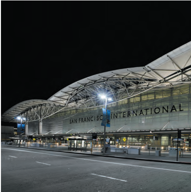
ROADWAY AREA LIGHTING
